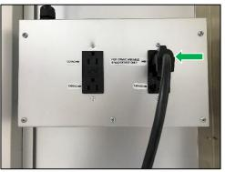
If the PAS750 unit is located inside the AG8000, plug the unit into the outlet labeled "FOR 120VAC VARIABLE SPEED DEVICE ONLY" as shown in the picture above.
