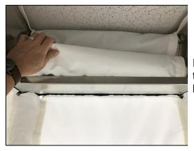
Roll up the top cover and place it in the cove in the header that is located opposite of the ladder.
