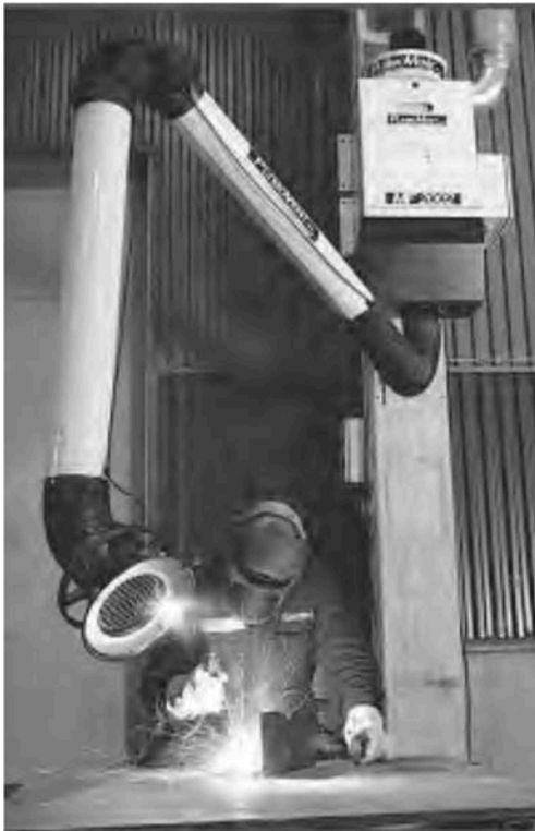
Figure 4: Source Capture Arm for Exhaust Ventilation. Courtesy Plymovent North America
