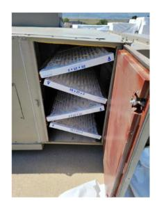
pre filter and a minimum MERV 13 final filter. If two stage filtration is not available, standalone or portable air cleaning units should come equipped with MERV 13 to HEPA filtration and be combined with UVGI for airstream disinfection. your filter supplier for proper maintenance and change out times depending on your facility.
